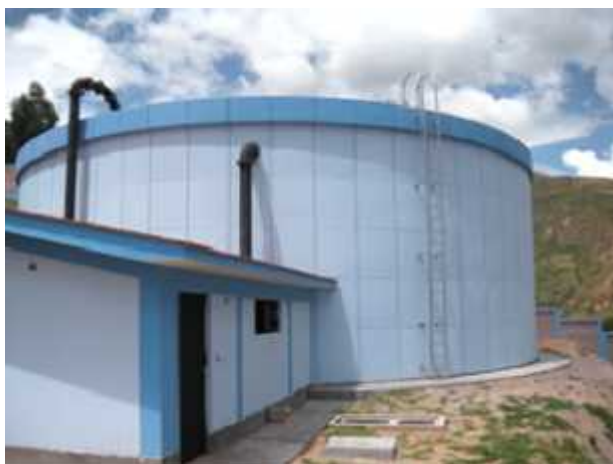
Reservorio de 1,500 m3, Huancayocc
